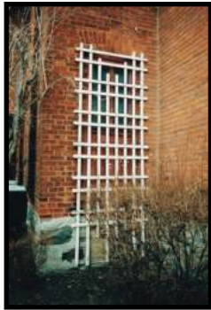
The trellis that hid an old boarded-up door was removed and a new white door now provides an easy access to the dining deck on the south side of the house.
