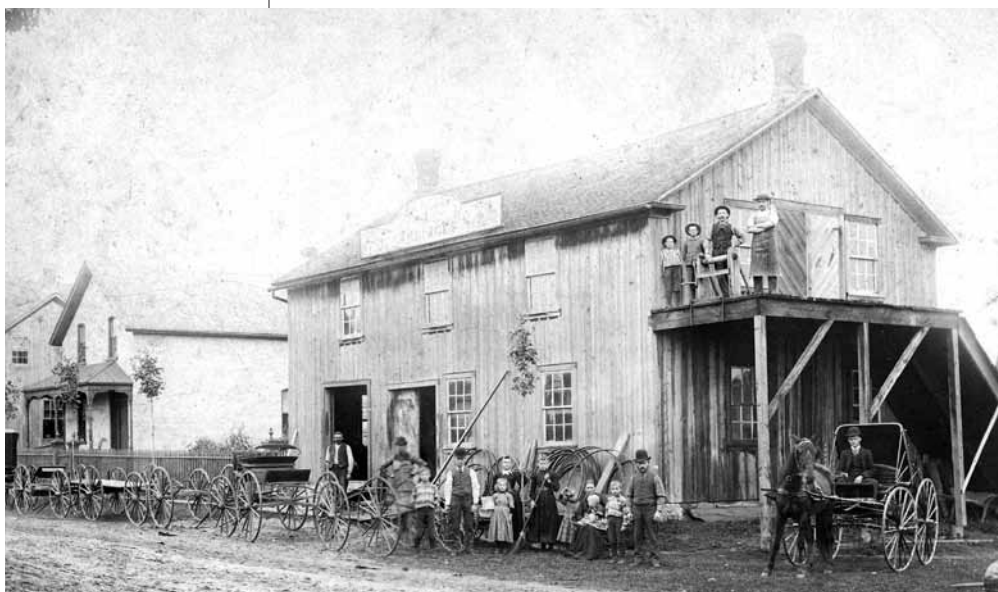
Above, the original carriage works established by William Matthies in 1874. The cover photo shows the Matthies Carriage Works with the new addition added in 1888.
