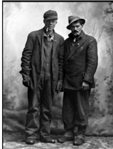
Unidentified labourers in work boots, coveralls, gloves and pipes in place. The man on the right is wearing two pairs of pants and his hat is cocked at such a rakish angle that it gives him a slightly roguish look.
